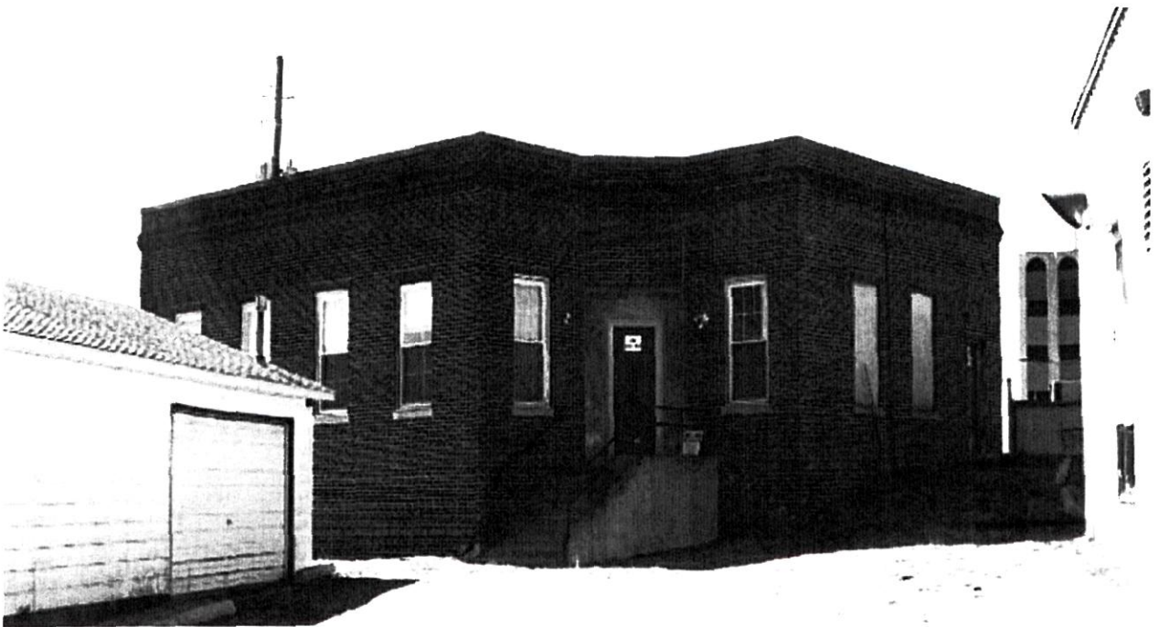
Peabody Coal Company Office, 2135 South 9th Street
