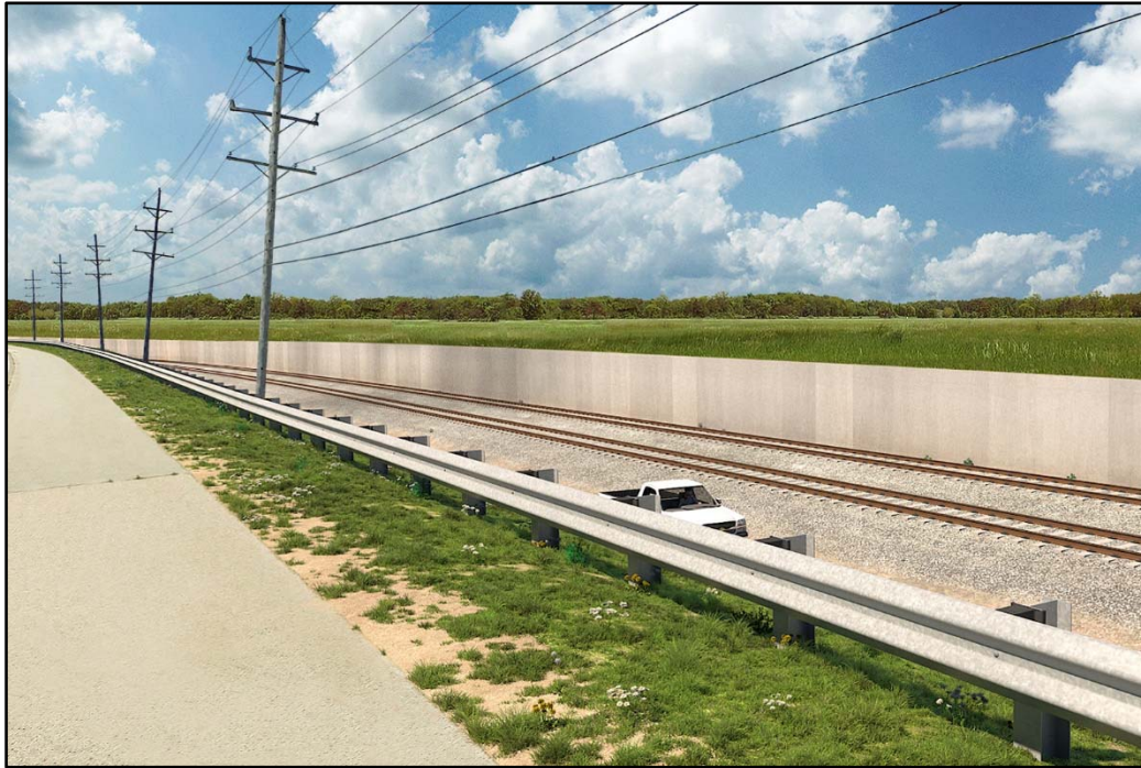
Figure 3-5. Rendering of Alternative 2A cut location with up to a 17-foot retaining wall west of UPRR (Station 2530+00)
