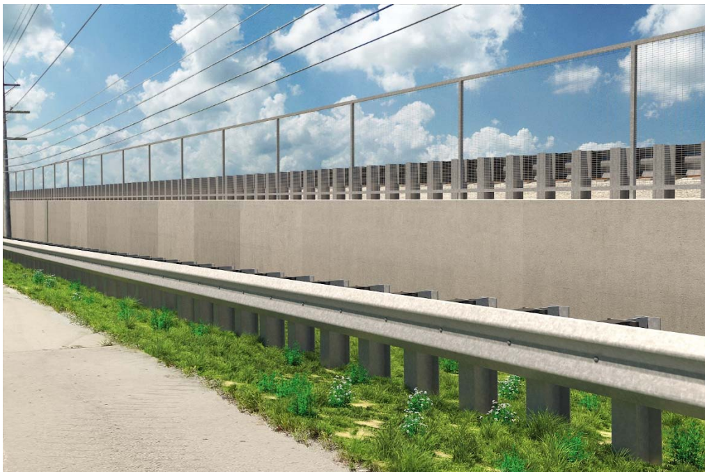
Figure 3-11. Rendering of Alternative 4A and 4B cut location with up to a 20-foot retaining wall east of UPRR (Station 2485+50)
