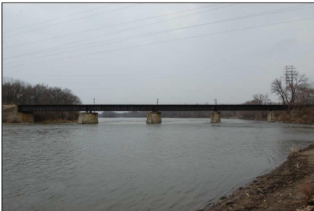
Exhibit 3-5. Kankakee River Bridge
