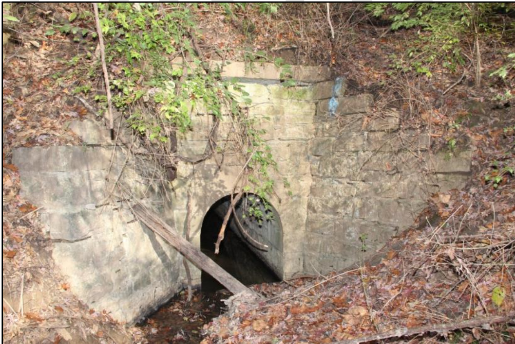
Figure 28: Located at MP 254.65, this stone culvert was constructed to facilitate drainage and the passage of water beneath the 1881 City of Alton bypass (Photo 7214).
