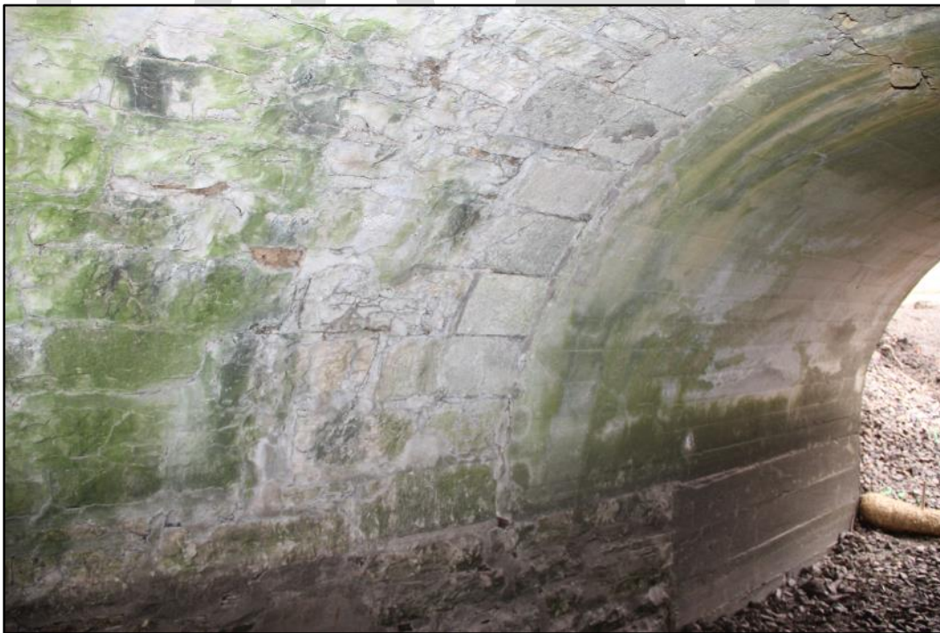
Figure 23: MP 163.60. Arch interior. Note the stone to concrete matching line (Photo 7130).
