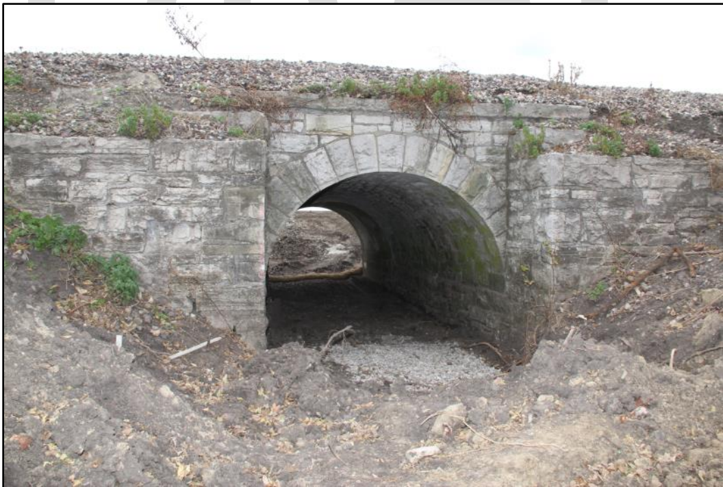
Figure 21: The east side of the culvert at MP 163.60 was constructed in 1876 of stone (Photo 7127).
