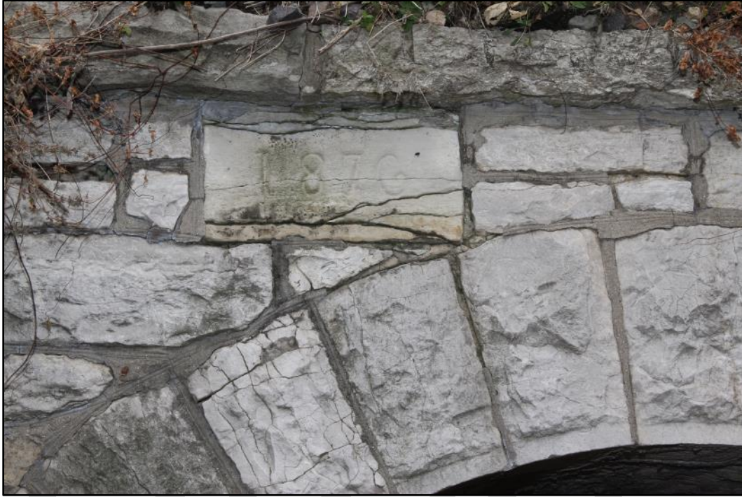
Figure 24: MP 163.60. 1876 date stone on the east side of the culvert (Photo 7126).
