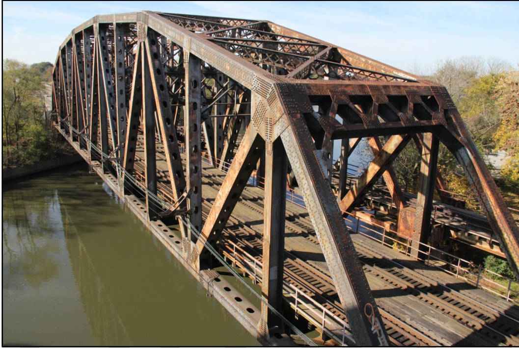
Figure 17: The only truss bridge located between Union Station in Chicago and Granite City, Illinois. Five similar bridges, on the Calumet SAG Canal immediately to the west have been documented for the Historic American Engineering Record (Photo 6933).
