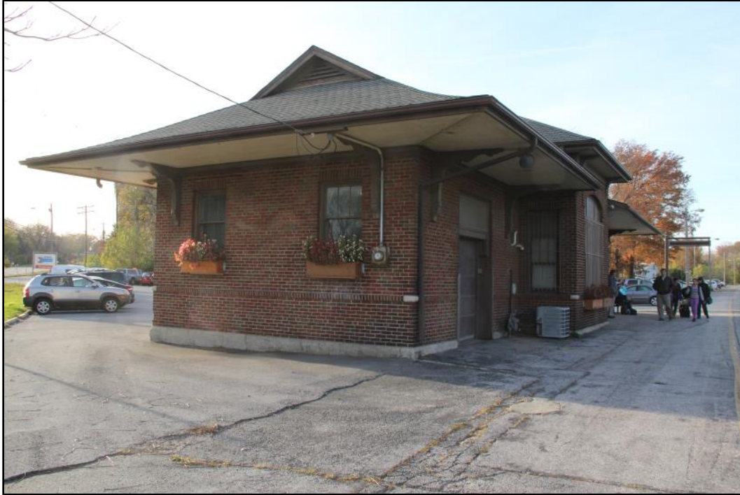
Alton Depot serves today both Amtrak and St. Louis commuter trains/Photo 7228
