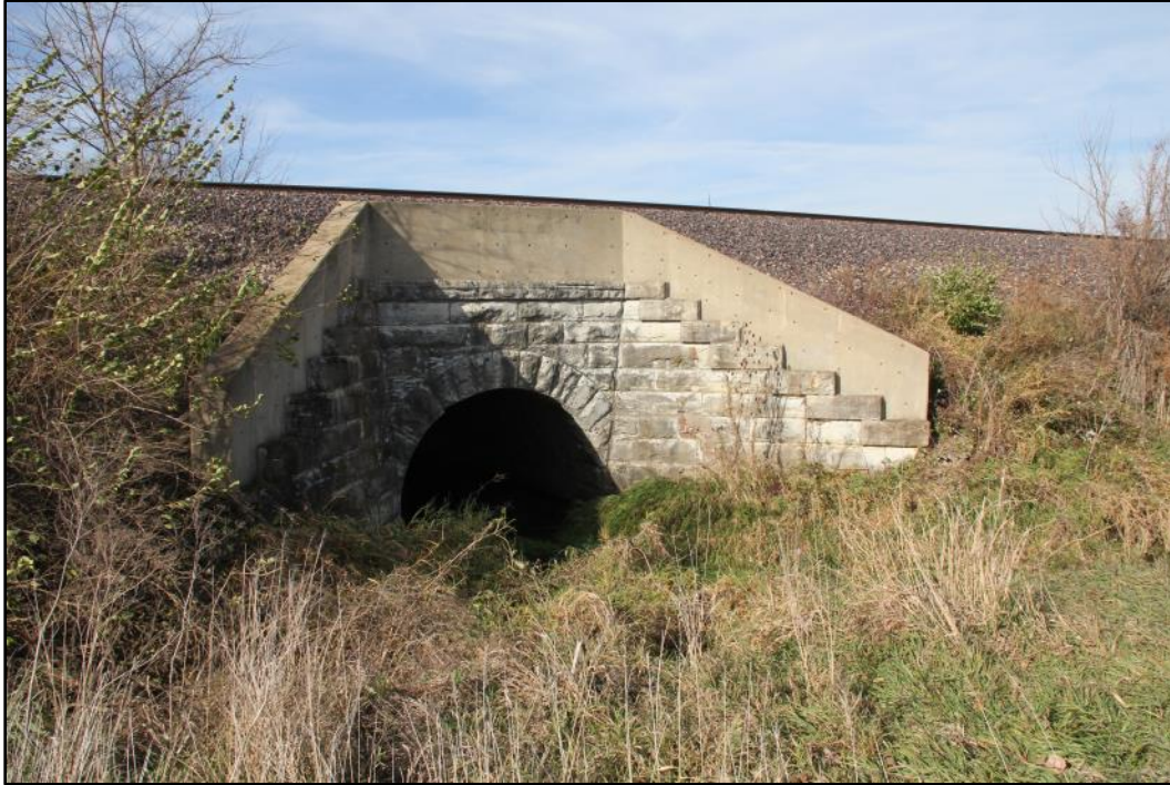
Figure 26: The east side of the culvert at MP 112.20 is likely the original. The segmental arch stones are finished and placed in a manner similar to the structure at MP 163.60. The retaining wall extension is a minor intrusion that is not thought to affect the overall integrity of the structure in a significant way (Photo 7249).
