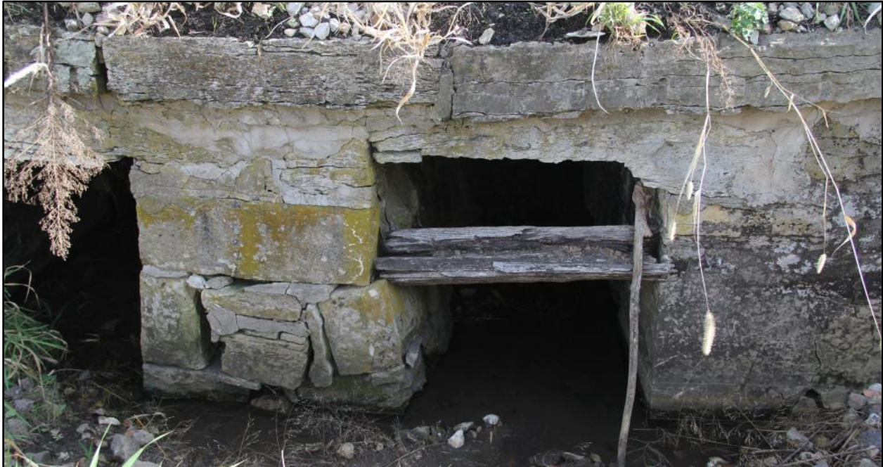
Figure 13: This small, two-opening structure located at mile post 46.95 (between Elwood and Wilmington) illustrates the second type of culvert noted.
