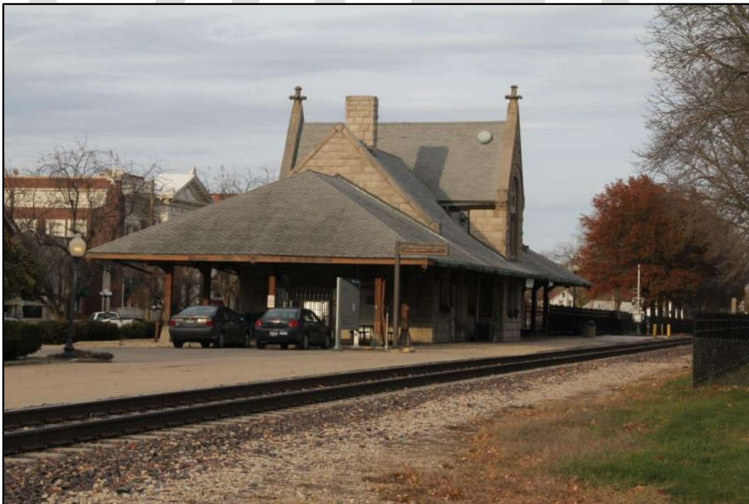
Dwight Station (National Register-Listed)/Photo 6986
