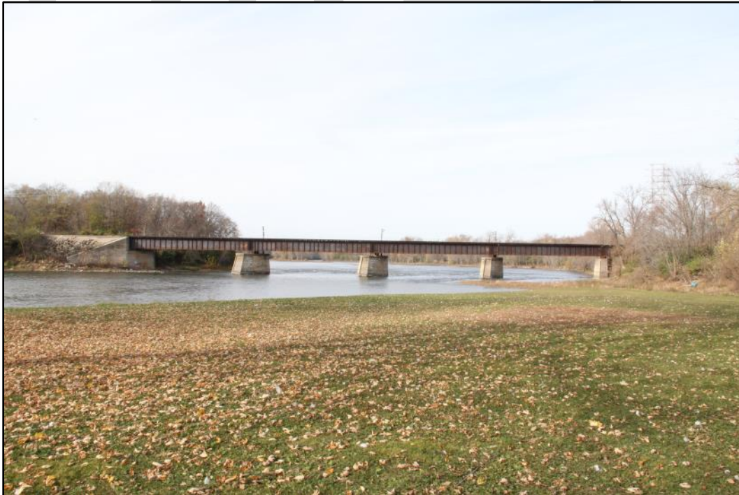
Figure18: Bridge over the Kankakee River in Wilmington (Photo 6964).
