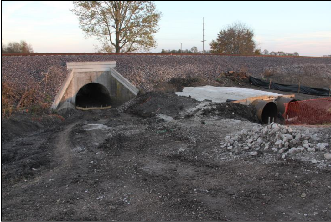
Figure 22: The west side of the culvert located at MP 163.60 was constructed of concrete, as often happened when a roadbed was being widened in the early twentieth century. A new, two-pipe culvert is presently being erected immediately to the southwest. Hopefully its construction does not mean that the original 1876 culvert will be removed (Photo 7097).
