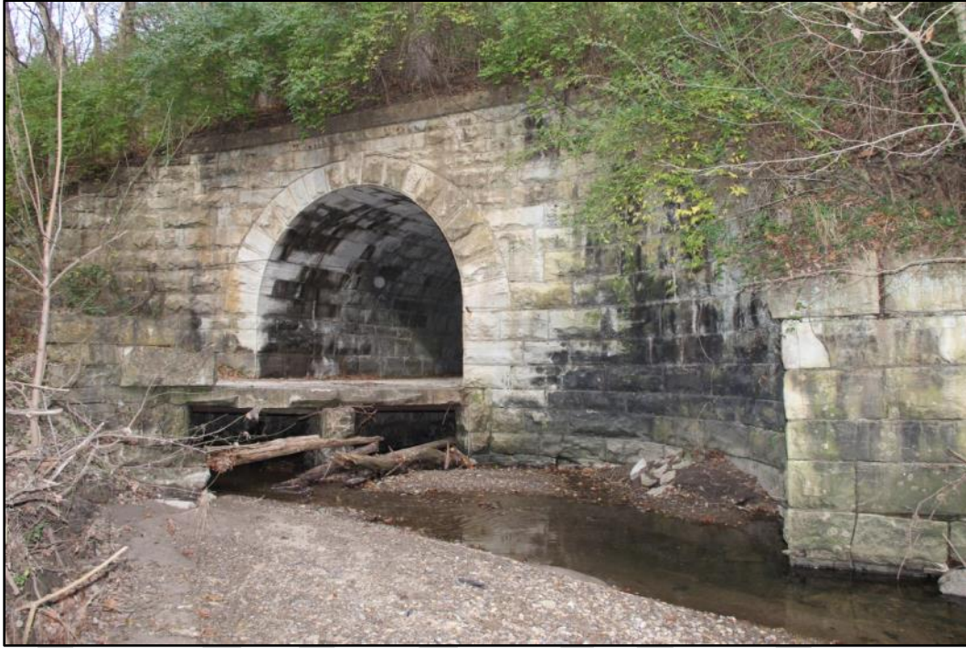
Figure 27: This very impressive, stone culvert is located at MP 254.30. It is located on the seven mile, City of Alton bypass and was constructed in 1881. It is presently being documented for the IL HAER recordation collection (Photo 7220).
