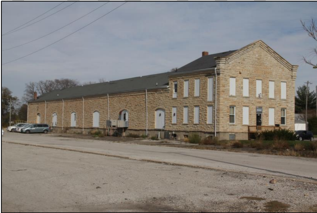
Chicago & Alton freight building adjacent to site of former Bloomington Shops/Photo 7060
