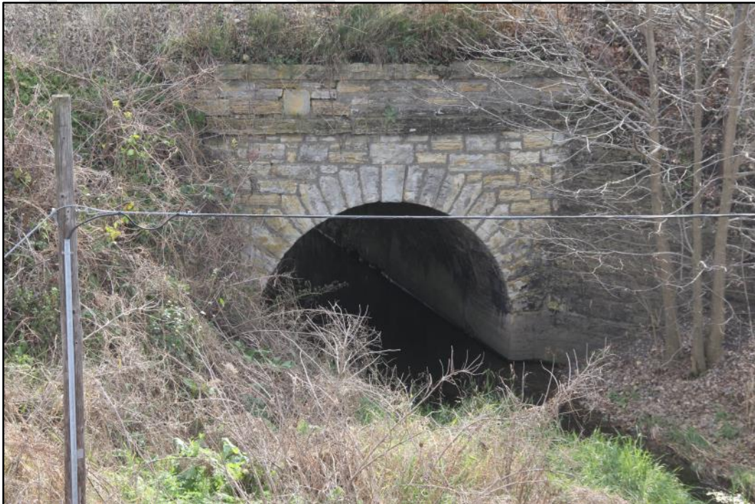
Figure 25: This is the west side of the stone culvert located at MP 112.20. This stonework is slightly different than that on the east side of the structure – which suggests it may be a bit newer. Nevertheless, this side of the structure exhibits significant character (Photo 7039).
