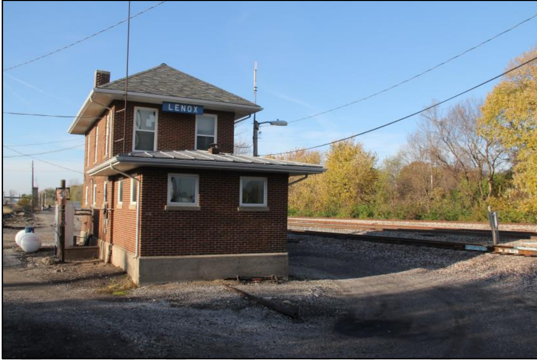
Figure 15: The Lenox Tower situated adjacent to the crossing of several railroads in Mitchell, Illinois (Photo 7245).
