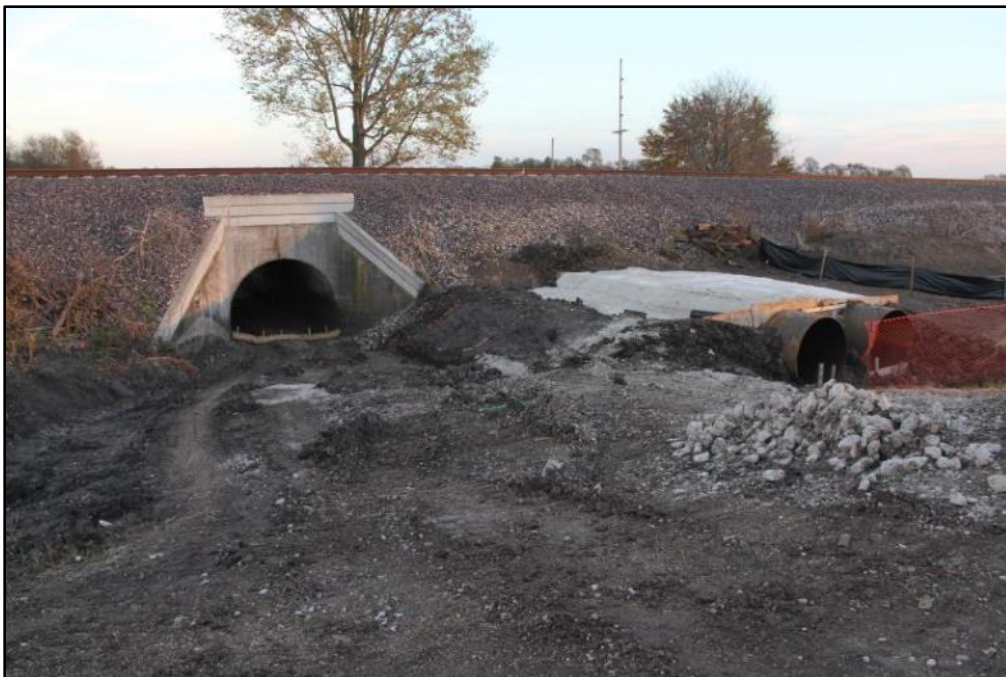
Figure 2: MP 163.60. Arched concrete side, view to east. Note new culvert adjacent.
