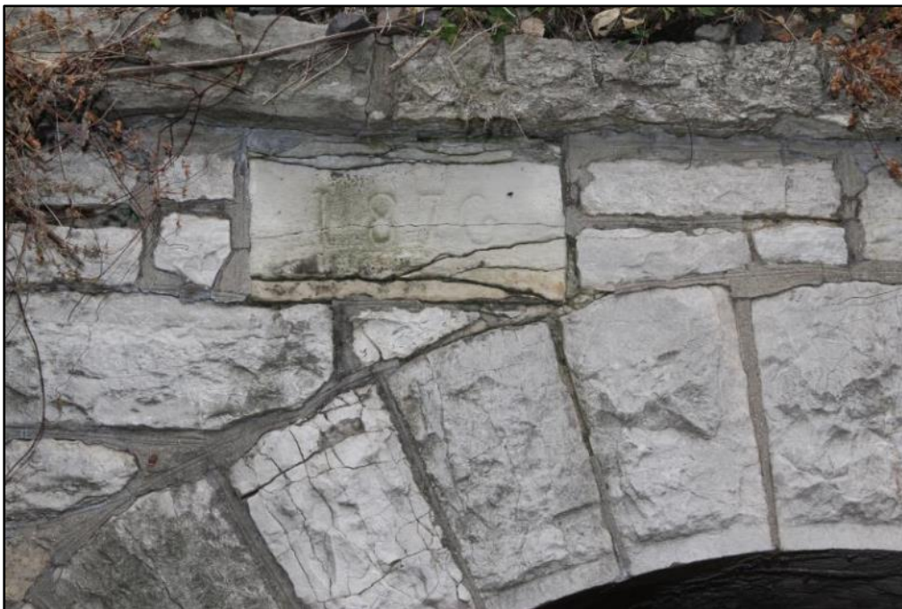
Figure 4: MP 163.60. 1876 date stone on the east side of the culvert.
