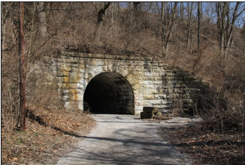
Figure 8: MP 254.30. View to east southeast. The consistent integrity of this substantial culvert structure is impressive.
