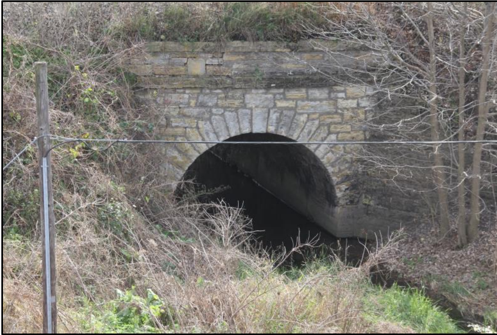
Figure 5: MP 112.20. View to east. This stone work (see the stones in the segmental arch) is slightly different than the stone work on the east side of the culvert—which suggests it may be a bit newer. Nevertheless, this side of the structure exhibits significant character.
