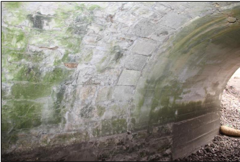
Figure 3: MP 163.60. Arch interior. Note the stone to concrete matching line.
