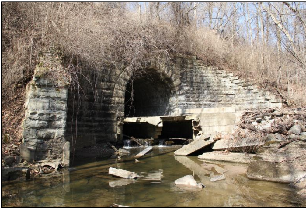
Figure 7: MP 254.30. View to northwest. With its dual capacity tunnel (two passage drain and roadway deck above), in addition to its excellent integrity, this is thought to be the most impressive example of late 19 th century stone work on the Chicago to Alton mainline.
