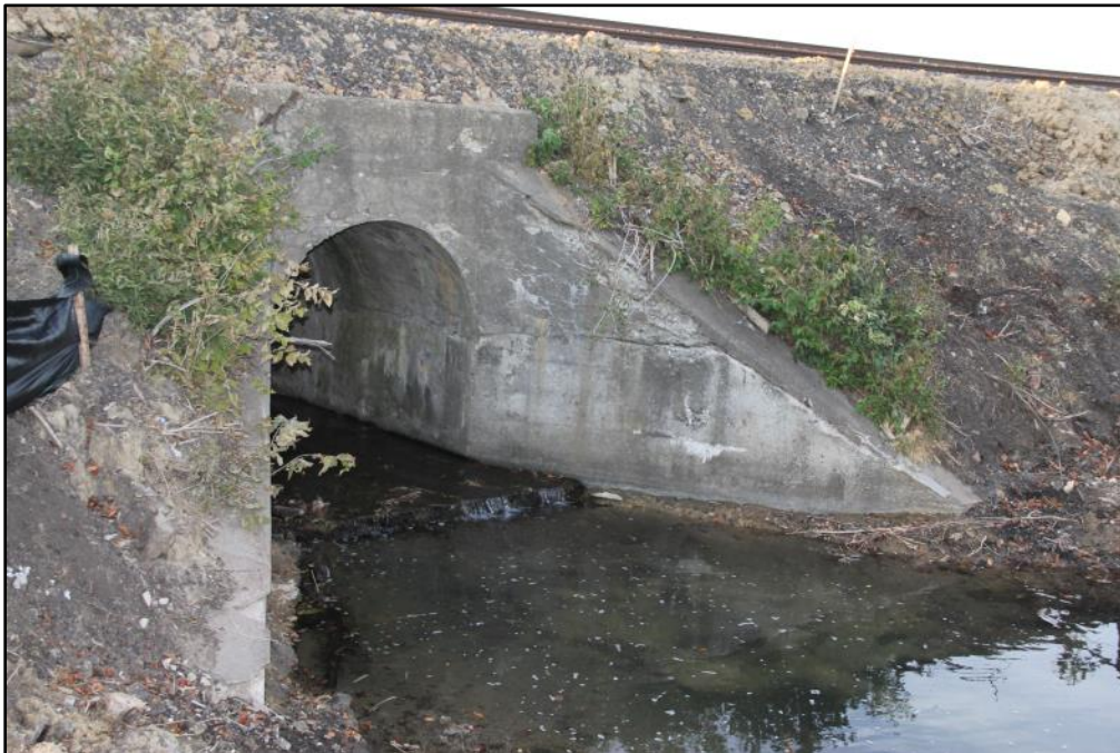
Figure 16: MP 162.70. View to northwest. It is unclear if this historic period culvert will remain once the installation of the new culverts is finished. Nevertheless, this is a relatively good example of a complete, concrete culvert that dates to the circa 1920 period.
