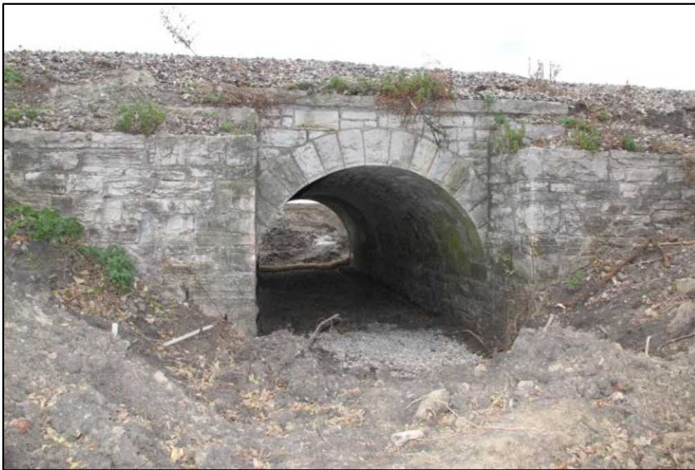
Figure 1: MP 163.60. Arched stone culvert side, view to west.
