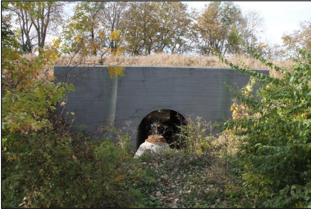
Figure 11: MP 127.10. Concrete culvert view to west.
