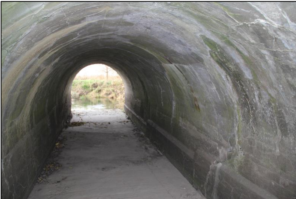
Figure 14: MP 152.70. Concrete culvert interior view to west.
