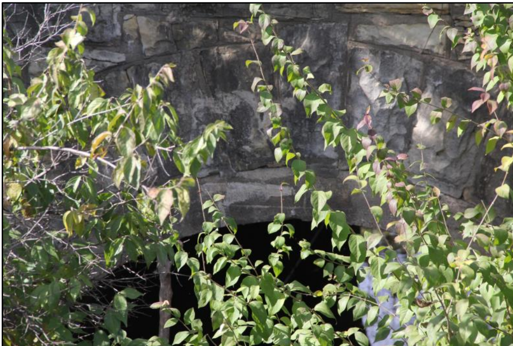
Figure 10: MP 47.30. View to west. Remaining foliage notwithstanding, it is apparent—as illustrated in this image—that the arch has been lined with a multiple inch thick layer of concrete, the date of which is unknown. But the addition of such a component significantly diminishes the integrity of the arch which is the key structural component of the culvert.
