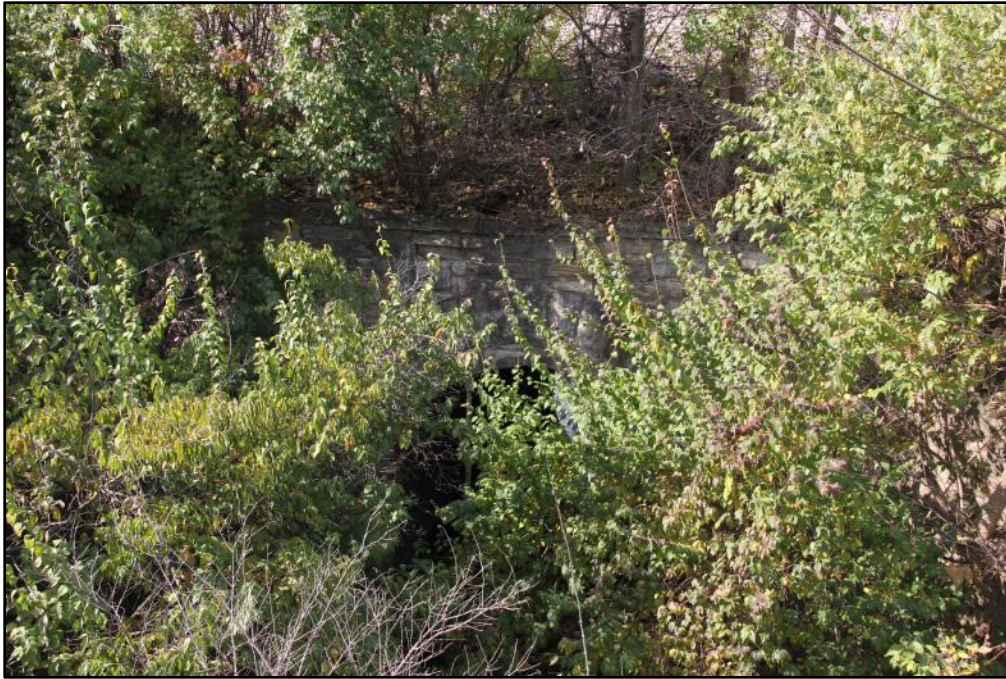
Figure 9: MP 47.30. View to west. The ability to view this structure well was obscured by the still apparent foliage.
