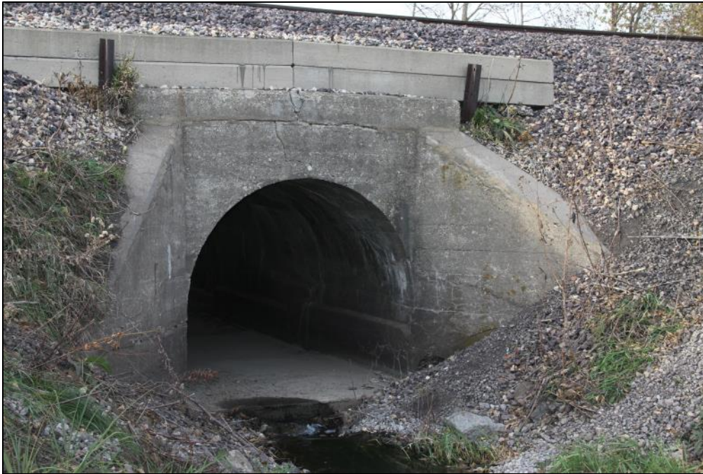
Figure 13: MP 152.70. Concrete culvert view to west.
