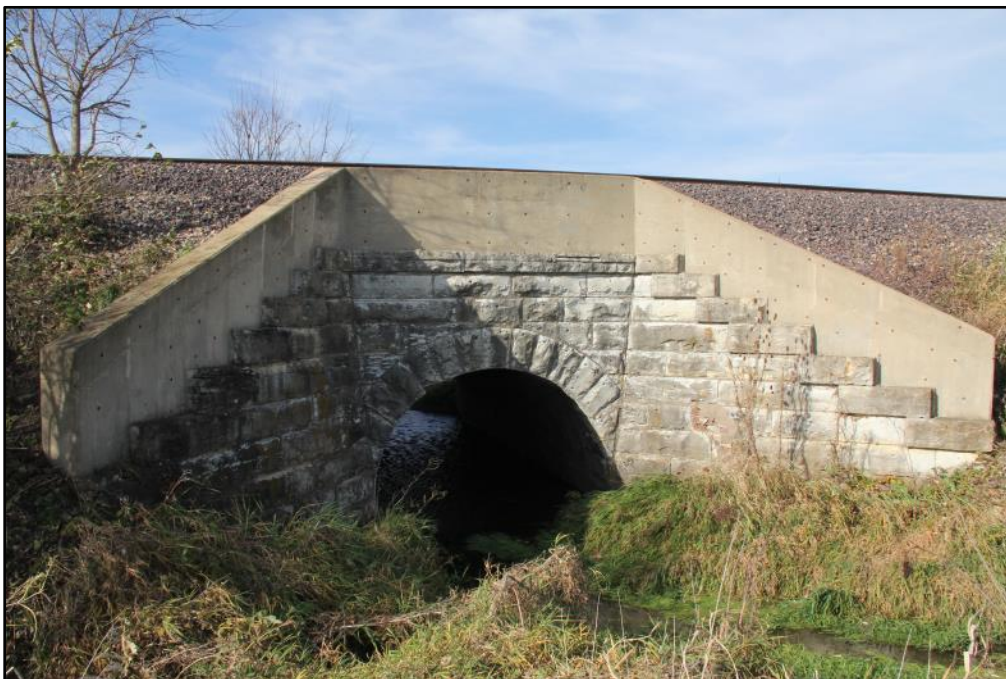
Figure 6: MP 112.20. View to west. This side of the culvert is likely the original. The segmental arch stones are finished and placed in a manner similar to the structure at MP 163.60. The retaining wall extension is a minor intrusion that is not thought to affect the overall integrity of the structure in a significant way.
