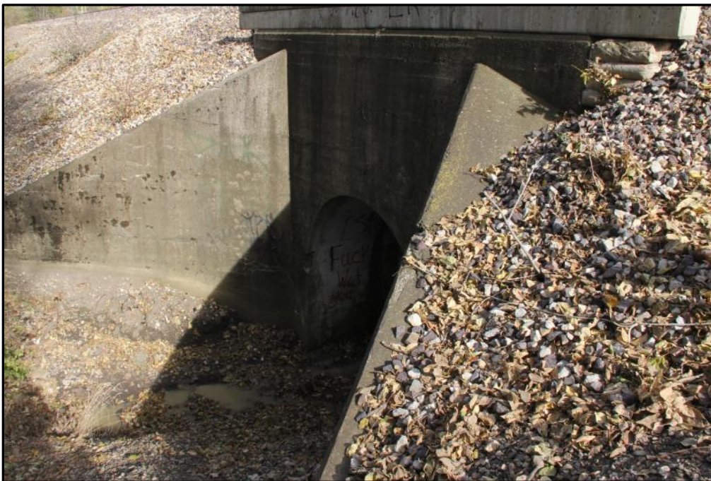
Figure 12: MP 127.10. Concrete culvert view to northeast.
