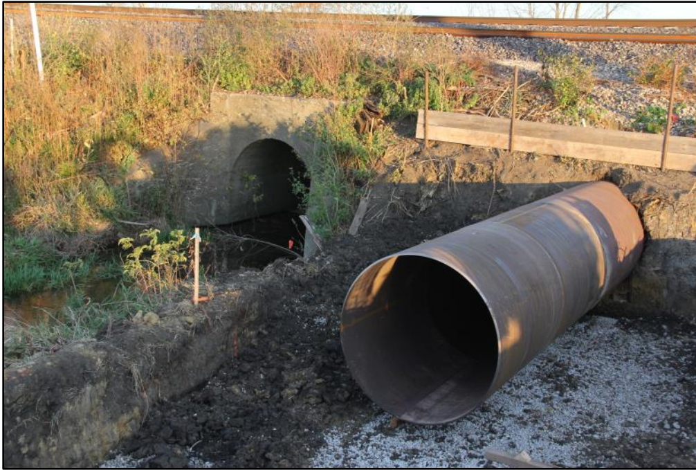
Figure 15: MP 162.70. View to east. New culverts are clearly being installed at this location.
